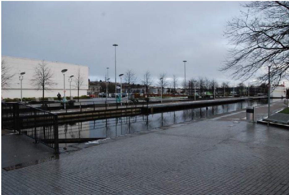
Figure 85 - Looking towards the North bank of the canal
