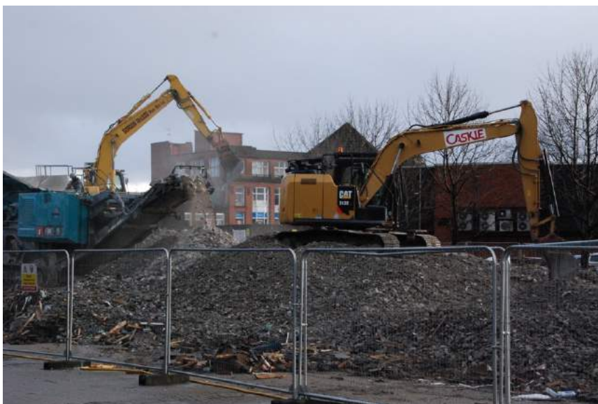
Figure 78 - Site clearance on Rosebery Place
